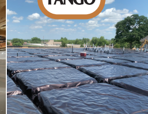
TERMITE AND VAPOR BARRIER
