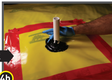
2 Cut an "X" the size of the pipe diameter in the center of the pipe boot and slide tightly over pipe.
