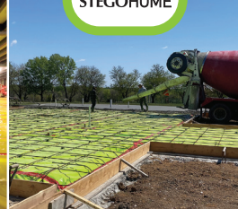
BELOW-SLAB VAPOR PROTECTION
