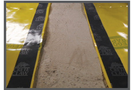
At a Location Designated by the Design Team: Install Stego Crete Claw onto the terminating edge of Stego Wrap.
