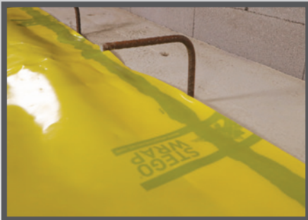
Onto a Perimeter Footing at Impediments: Seal Stego Wrap to concrete with Stego Mastic.
