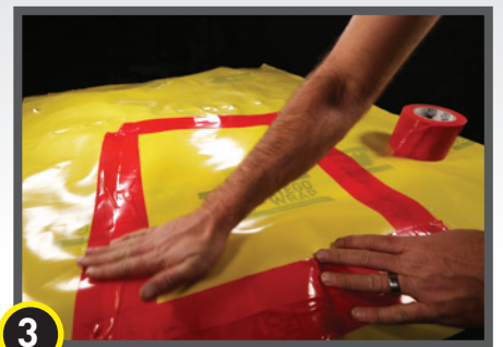
3 Measure and cut a piece of Stego Wrap to cover damaged area 6" in all directions. Seal patch with Stego Tape.
