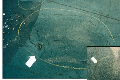
Figure 3. A typical blistered area of a swimming pool coating was 15 inches in diameter (top). Overnight, blisters collapsed and receded in diameter while visible moisture in the blisters appeared to dissipate (right).
