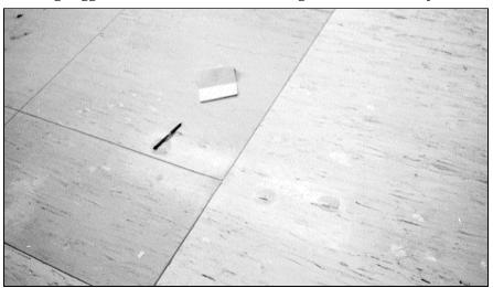
Figure 2. Blisters in seamless vinyl flooring are commonly caused by moisture emissions in concrete floors. Most blisters in this hospital surgical suite ranged from 1 inch to 4 inches in diameter.
