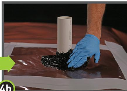
**4b** Seal around the base of the pipe with Drago Mastic. Note: apply using disposable glove, paint brush, or similar.
