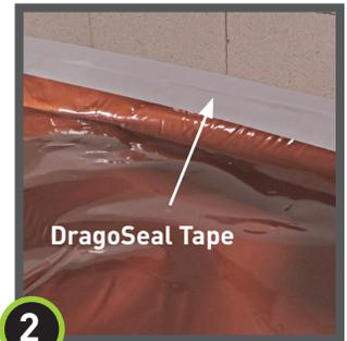
Apply **DragoSeal Tape** on the perimeter edge so that 2" is on the Drago Wrap and 2" is on the wall/vertical surface. Press firmly to secure.
