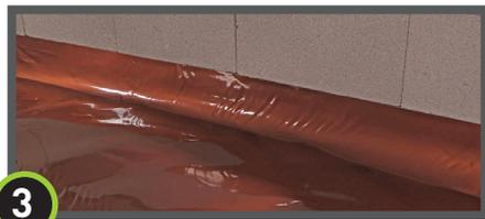
Press Drago Wrap firmly against **DragoTack Tape** to secure.
