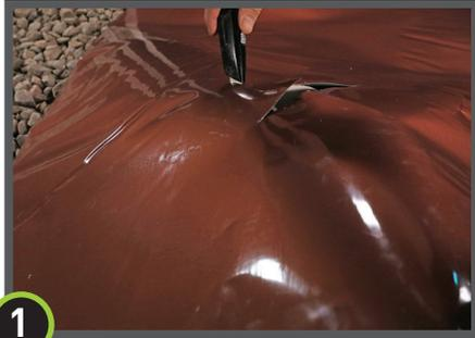
**1** Install Drago Wrap around pipe penetrations by slitting/cutting material as needed. Try to minimize the void space created.
