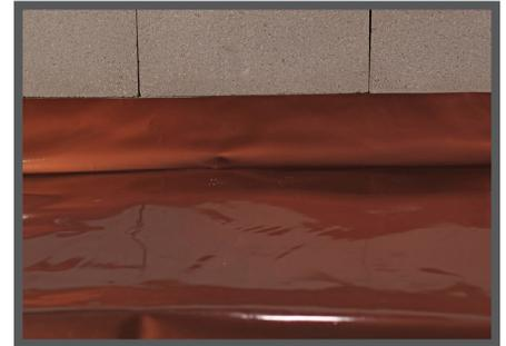
Note: Turn Drago Wrap up foundation walls or forms. Ensure Drago Wrap is flush against the corner to avoid tenting.
