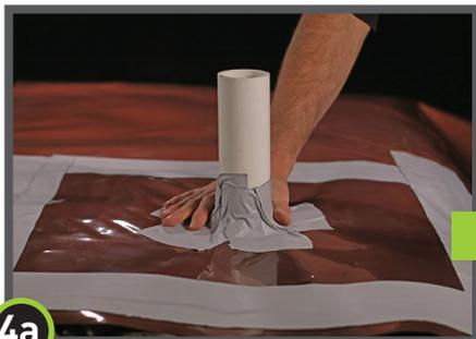
**4a** Seal around the base of the pipe using DragoSeal Tape.
