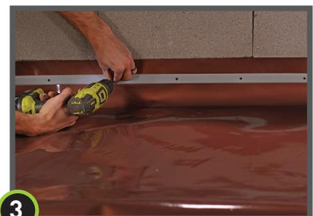
Fasten a termination bar over the top of the Drago Wrap in line with the Drago Mastic.
