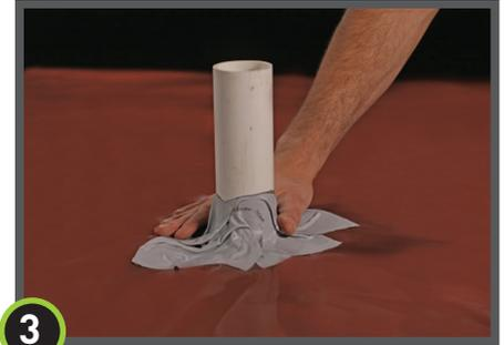
**3** If Drago Wrap is close to pipe and void space is minimized then seal around pipe penetration with either DragoSeal Tape (as shown), Drago Mastic or Drago Sealant and Drago Sealant Form.
