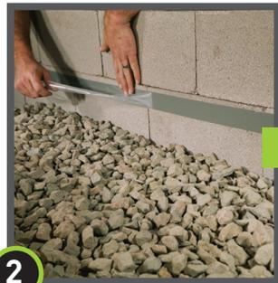
When ready to apply Drago Wrap, remove the exposed release liner from **DragoTack Tape**.
