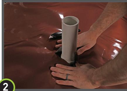
**2** Pull material over and flatten. Clean area of adhesion where the Drago accessory will be applied.
