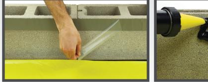
Make sure area of adhesion is free of dust, dirt, debris, moisture, and frost to allow maximum adhesion.
