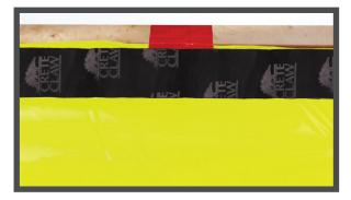
Extend Stego Wrap to the height of the slab (likely the height of the forms).
