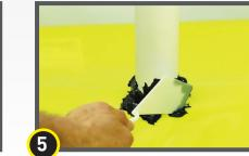
If Stego Mastic is applied unevenly at first pass, it can be evened out with a trowel or by hand
