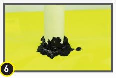
Completely sealed pipe penetration
