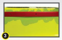
Utilize Stego Term Bar or other means (e.g. concrete, backfill) to provide consistent, continuous pressure to the Wrap-Mastic interface
