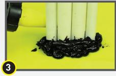
Stego Mastic should completely seal the edge of the wrap to the penetrations
