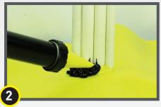
Where multiple pipes are close together, place mastic around and between all individual pipes
