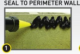
Apply Stego Mastic liberally (~2 inch width and minimum 60-mils depth) behind where Stego Wrap will terminate
