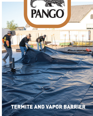
BELOW-SLAB VAPOR AND RADON GAS PROTECTION
