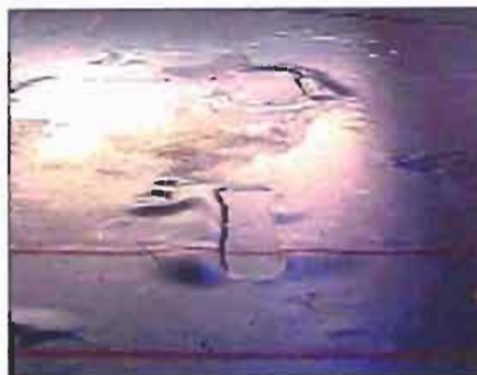
Moisture can have a devastating effect on floor coverings, such as this failed gym floor.
