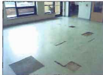
A vapor retarder placed under granular fill may trap rainwater, leading to such moisture problems as were later seen with this tile floor.
