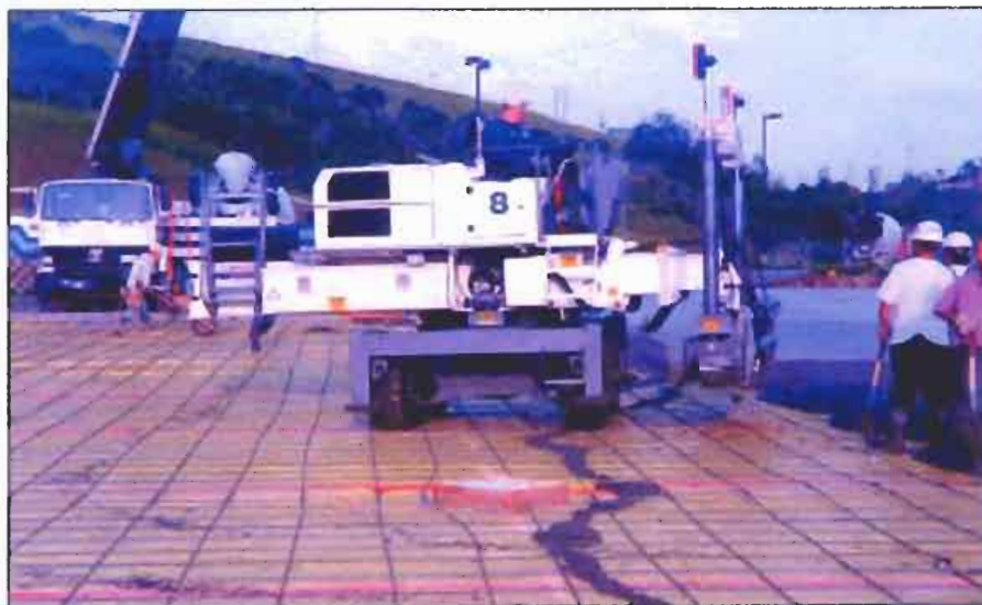
A thicker vapor barrier is required where there will be equipment traffic or with angular base materials. Note the example of torn 6-mil poly.
